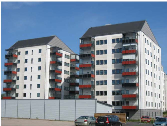
Passive houses in Växjö
