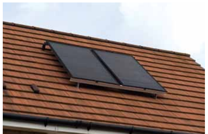
Figure 2. A flat-plate system
