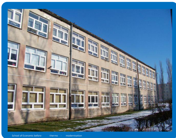
School of Economic before thermo - modernisation
