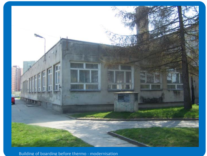
Building of boarding before thermo - modernisation
