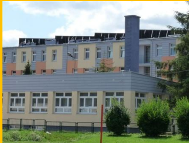
Building of boarding after thermo modernisation
