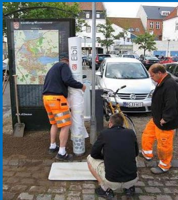
Placing a charging point in Kolding, Triangle Region, Denmark 2011
