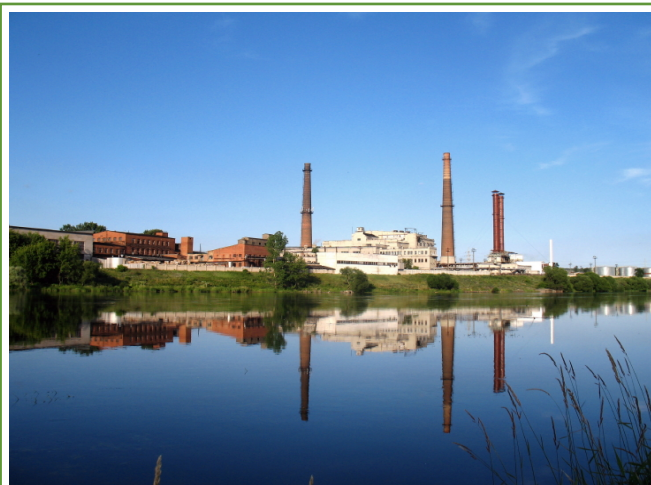
Petrašiūnai power plant, to be converted to biomass by 2015. Kaunas Region (Lithuania), © AB Kauno energija.
